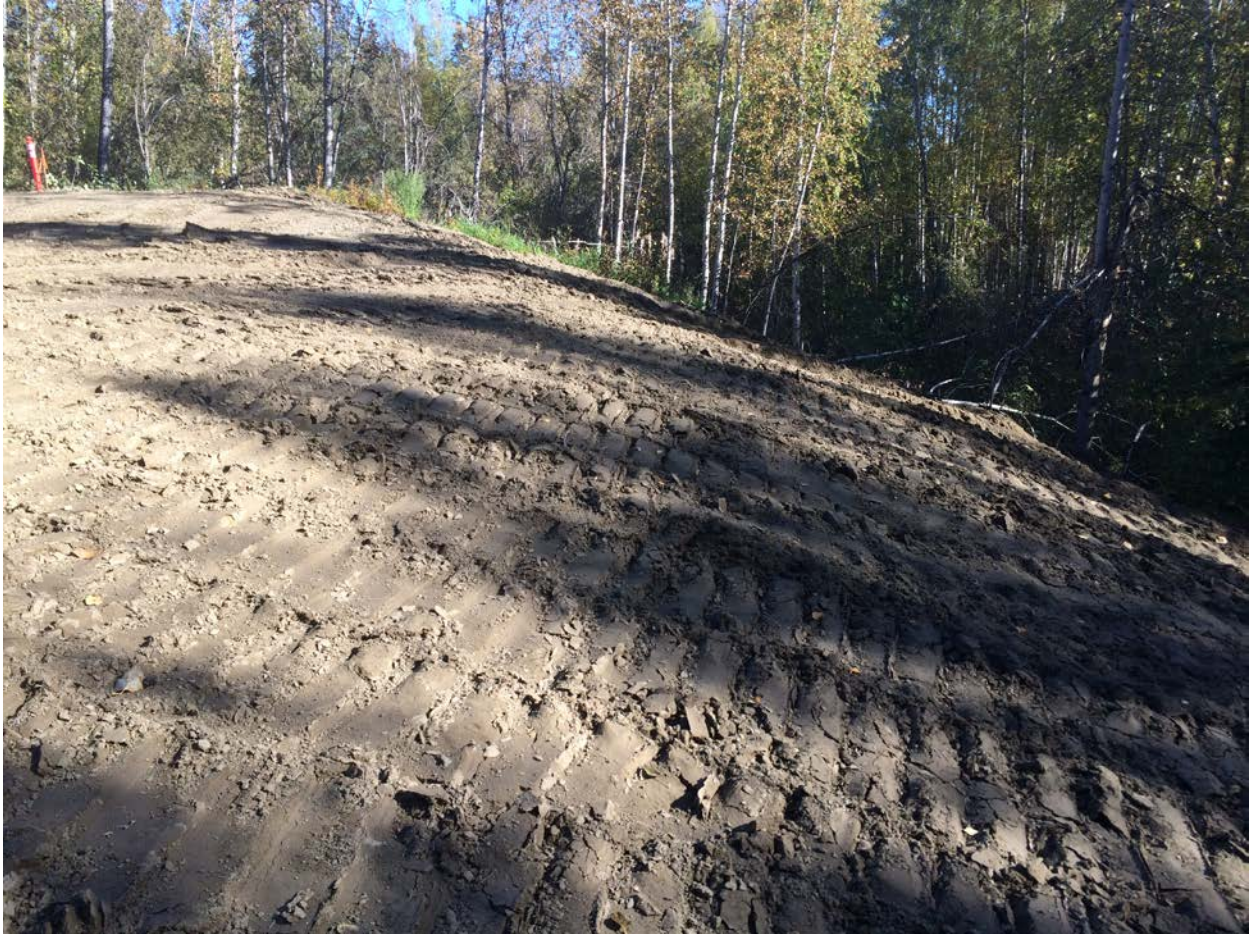
Figure 2 - Graded slope at the south of the site.
